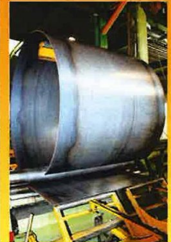
Tank rolling in progress
